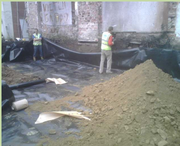
The insertion of the GeoTextile Membrane
