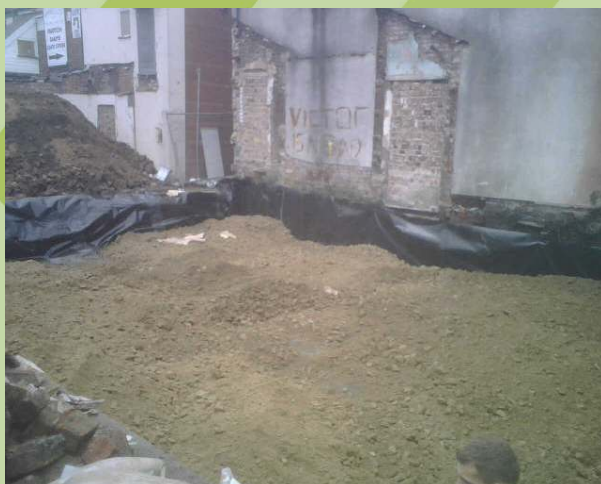
The backfill and compaction of the excavated area
