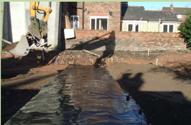
The membrane in place before the ground is stabilised
