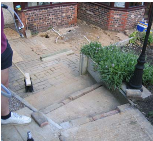
Wells Installed and awaiting paving
