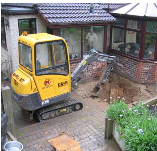
Hydrocarbon Affected Areas
