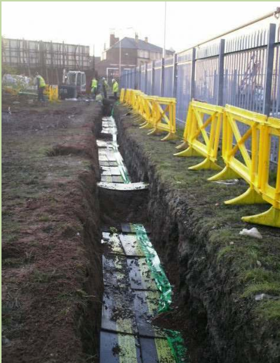
New service trenches to the substation
